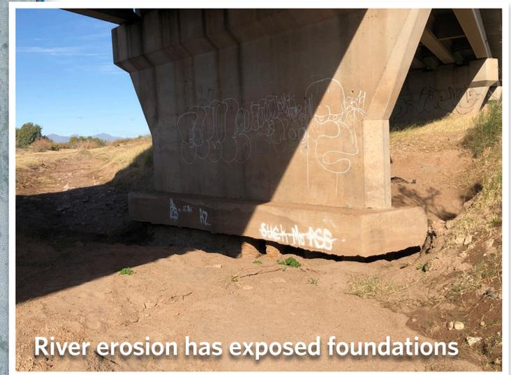
River erosion has exposed foundations
